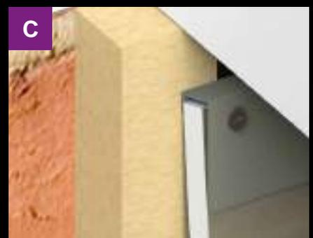
**End Closure Profile:** To finish Dura Cladding Resist where installed in a lap configuration.
