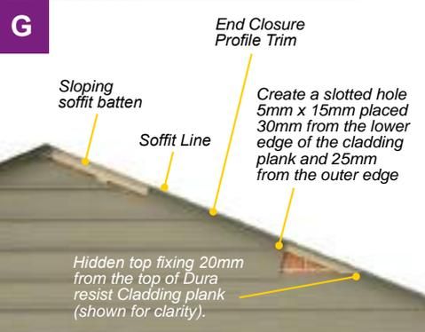
On a gable end with a triangular abutment, the Dura Cladding Resist plank needs to be fixed at the top and bottom to the batten which runs parallel to the roof slope. Failure to secure the bottom edge can result in the curling of the plank in certain conditions.
