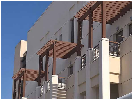
Dura Pergolas in verandas at SEG Doha University Campus
